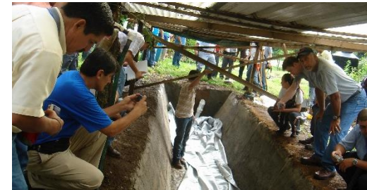
Installing a tubular biodigester. Inception meeting of the RedBioLAC, Costa Rica 2010
