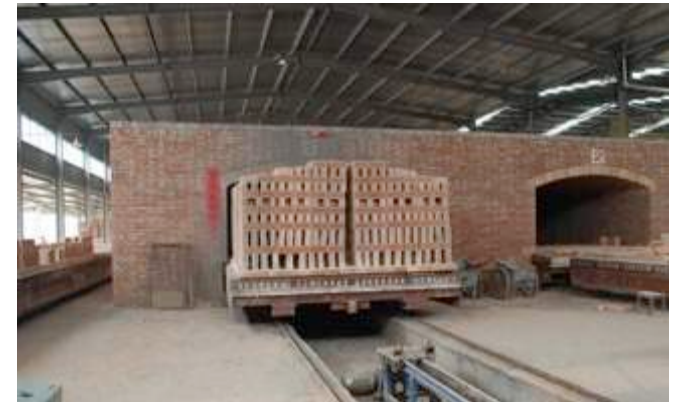
Financed 6 energy efficient Auto-brick projects
