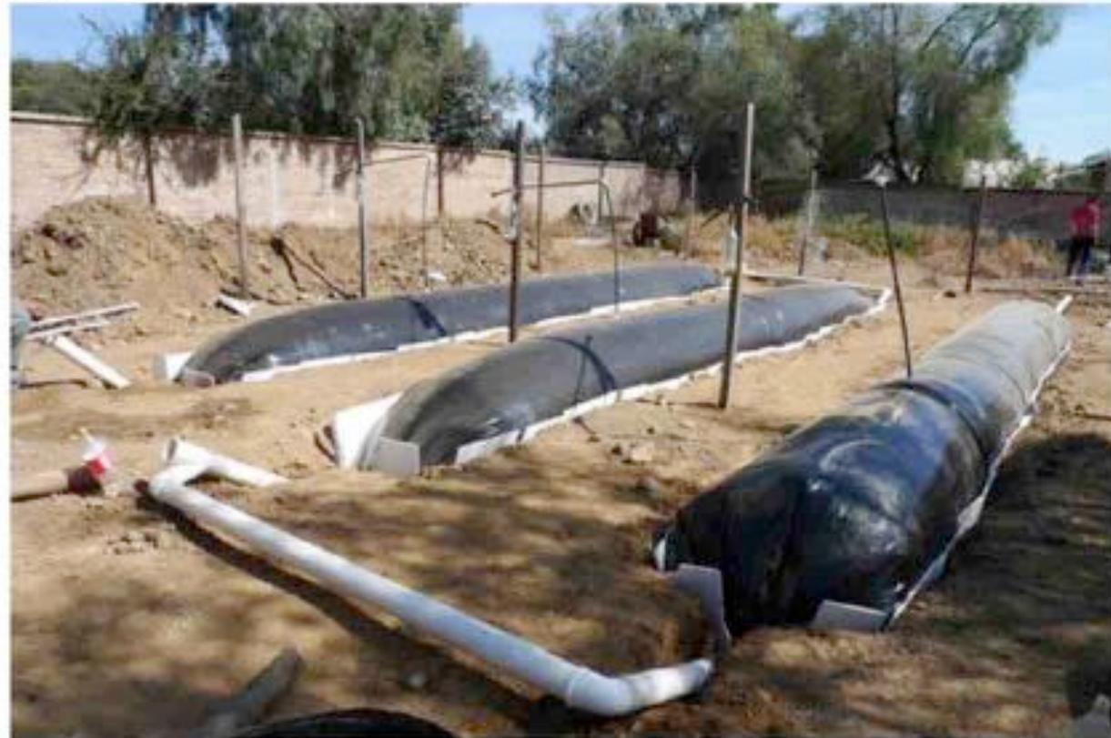
**Fig. 1.** The three tubular digesters in series, monitored in the Cochabamba slaughterhouse, at 2572 m above sea level (Martí-Herrero et al., 2016).
