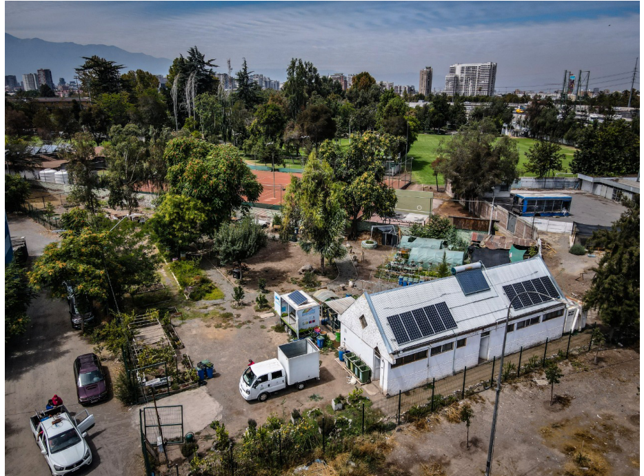
Community Energy Centre by the Municipality of Independencia
