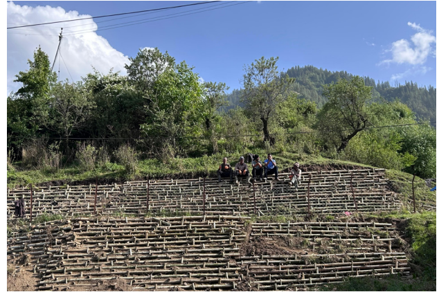
After Installation of Crib Wall
