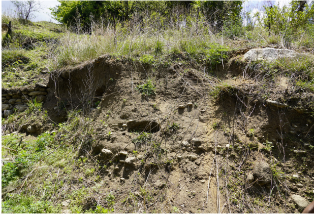
Slope before Installation of Crib Wall
