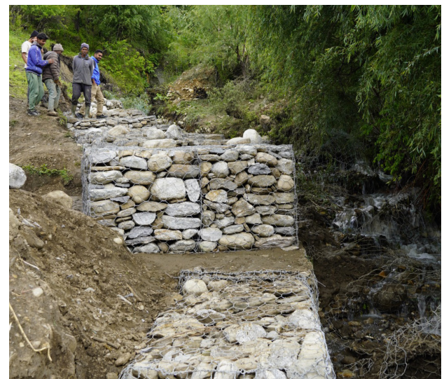
Condition after installation of gabion walls
