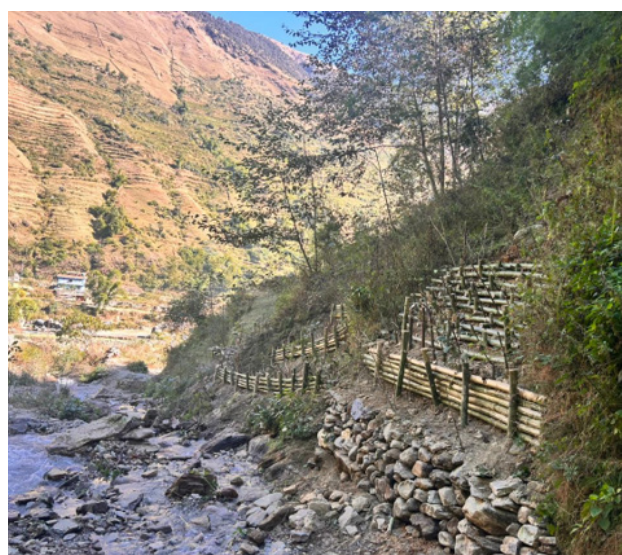
Bioengineering on the riverside of one of the streams flowing beside the powerhouse
