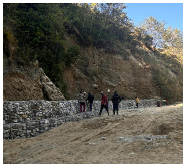
Gabion walls installed for landslide protection above the powerhouse
