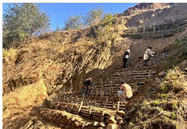
After intervention: Dry stone walls, Bamboo Retaining wall and Bamboo Crib walls are constructed
